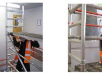
8. Climb partially through the second trapdoor platform and adopt the 3T position as in 6. Fit four 1.5M horizontal guardrail braces to the verticals of the frames 0.5m and 1.0m above the platform frames to either end of the tower. Fit a second trapdoor to make a guard rail and then fit a diagonal brace to continue the platform at the level of the top rung on the ladder frame zig-zag bracing pattern. The brace should be placed on the flush side of the platform.
