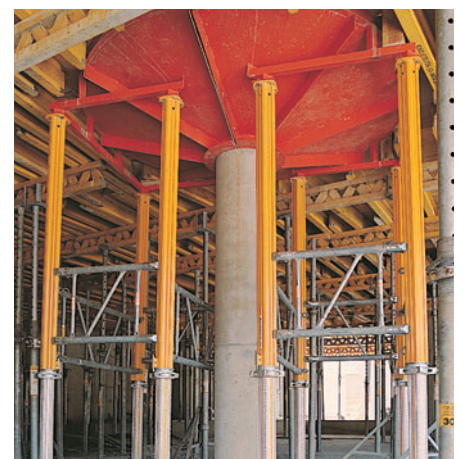
MP 350 with frames supporting column capital formwork.
