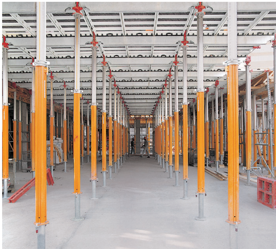
MULTIPROP 350 with Base MP 50 together with SKYDECK being used to shutter a slab with a clear height of 4.10 m.
