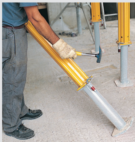
The Base MP 50 can be fixed quickly. The quick-action clamp coupler makes it possible.
