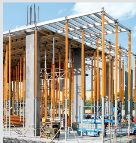
MRK frames can be used to brace high MULTIPROPs.
