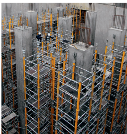
MULTIPROP towers with working platforms as shoring system for any height.
