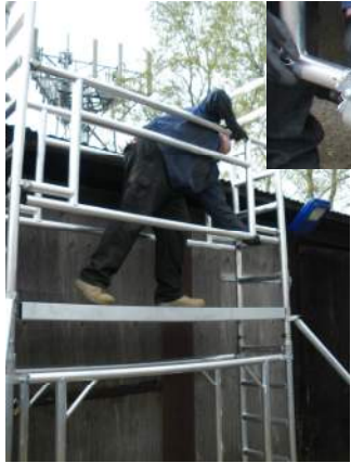
7. Ensure all clamps are locked.
