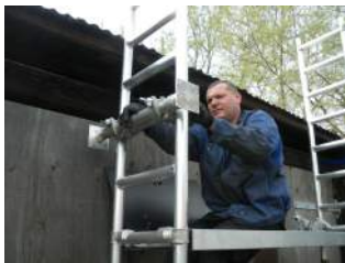
8. Fit next upper frames on to base frames and ensure clips are located in spigot holes.
