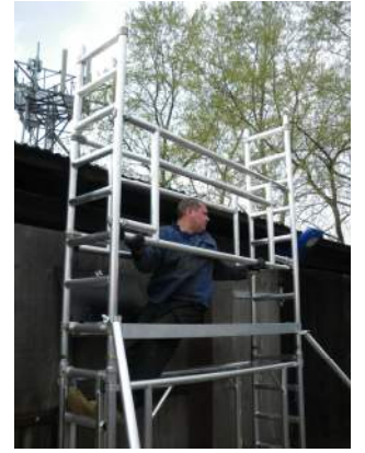
6. From a sitting position fit the handrail frames
