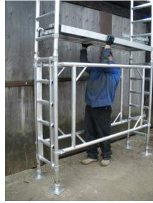
5. Fit opposite frame and locate the platform on rung shown.
