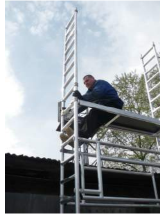
10. Fit next frames and lock clips, fit brace frames.
