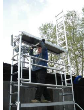
9. Fit next platform on 8th rung of frame above platform.
