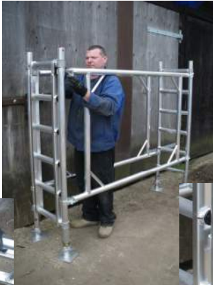
2. Fit opposite guardrail brace frame and level unit using adjustable legs.
