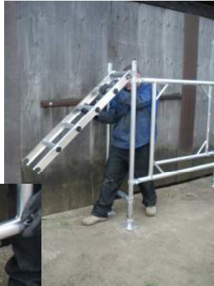
3. Access is through end ladder.
