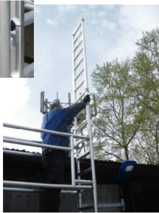
8. Fit next upper frames on to base frames and ensure clips are located in spigot holes.
