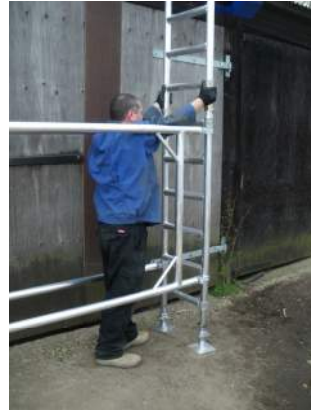
4. Fit next frame on one end
