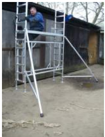
7. Ensure all clamps are locked.
