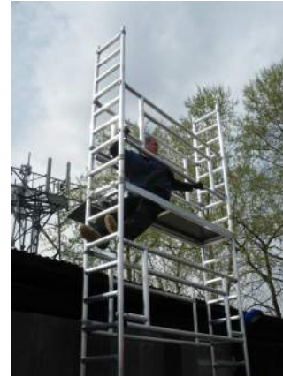
10. Fit next frames and lock clips, fit brace frames.
